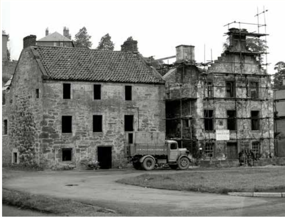
Houses at Sandhaven, Culross being restored (1958) © NATIONAL TRUST FOR SCOTLAND
