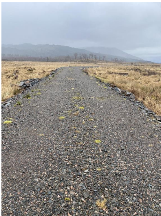
Plate 5: Floating track bisecting the Site.
