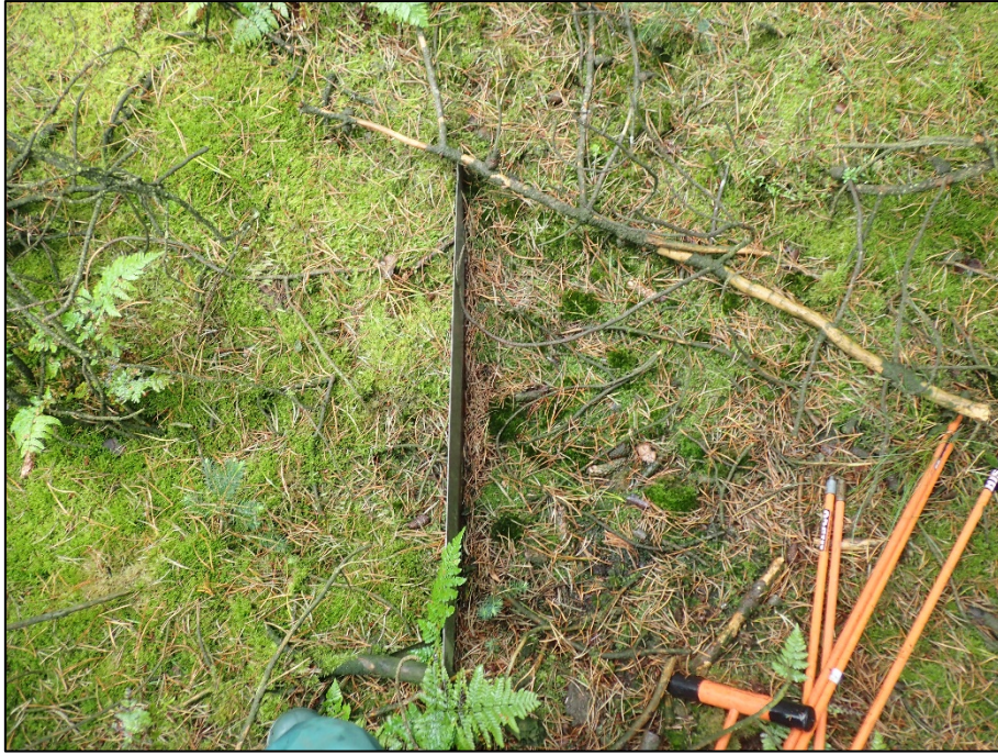
Figure 3: Plastic piling successfully blocking a ditch on site and encouraging sphagnum regeneration.
