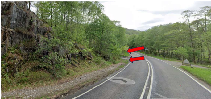
Figure 21 Entrance/Exit to old road loop
