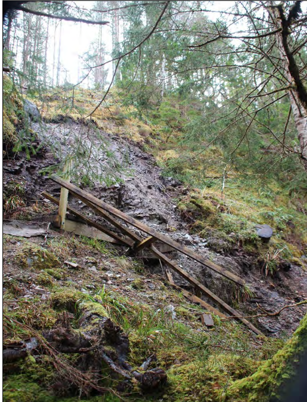
Damage to the recreational infrastructure caused by a storm in January 2015. Ravens Rock. Photo: A. Baranska, NHFD
