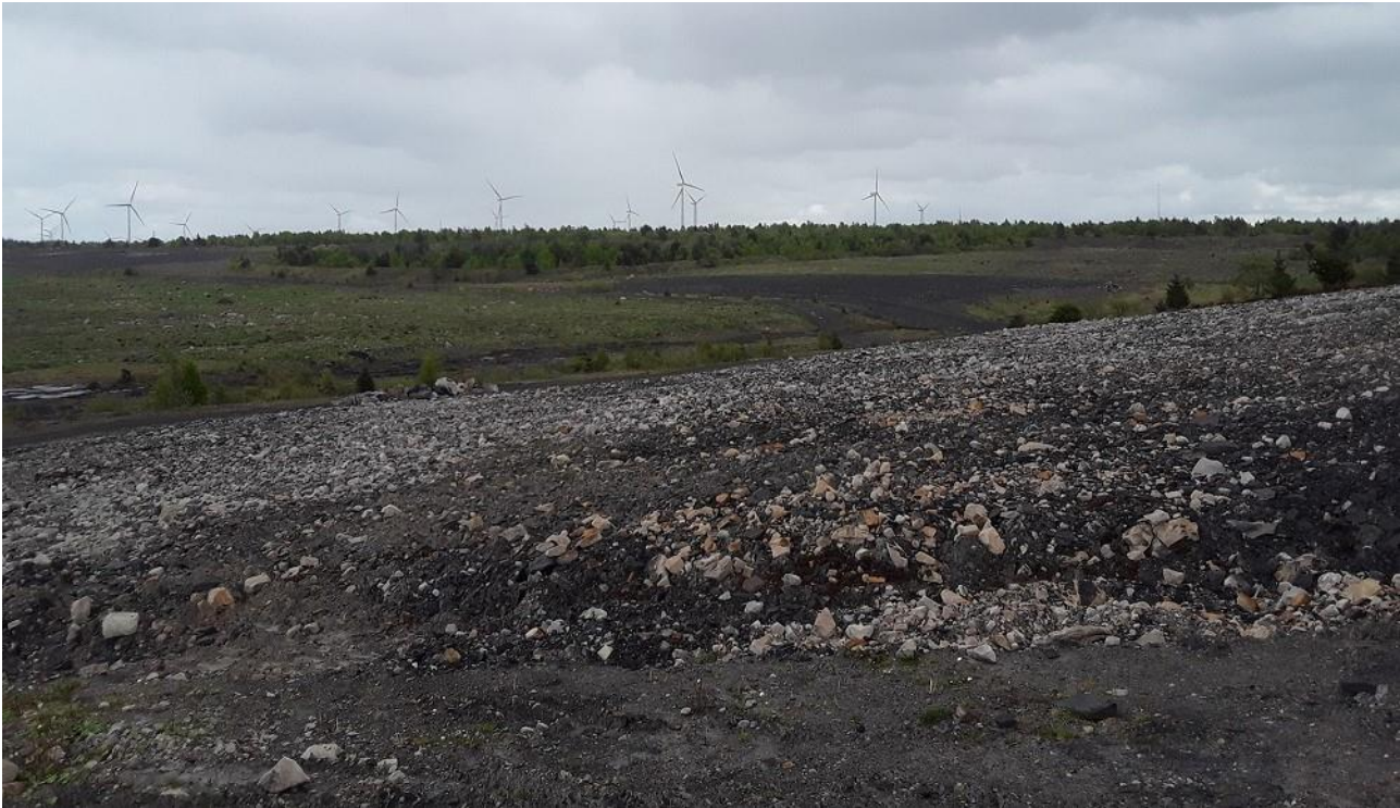
Picture 1: A typical view across recently remediated former mining ground at Damside. Man-made soils are of mixed clay and coarse stone, enriched and mechanically de-compacted.
