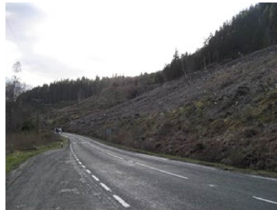
Steep slope felling operations create large scale and dramatic change over the short term
